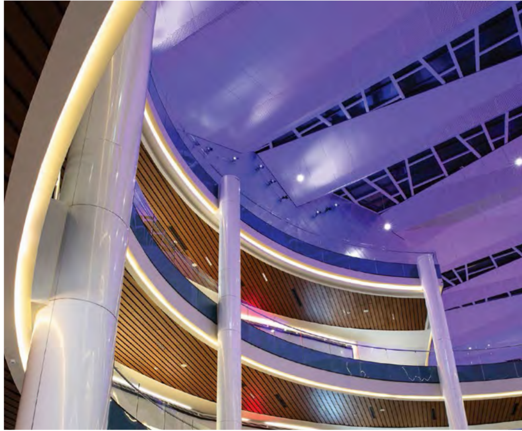
Fashion Drive shopping centre Monterrey, Mexico 2018 Finish: Golden pearl Material: Stacbond FR System: Ad-hoc Transformation: Bending with rollers
