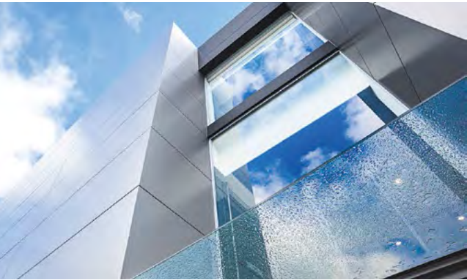
Porsche Car Dealer A Coruña, Spain 2017 Finish: Silver metallic Material: Stacbond FR System: STB-CH Transformation: Bending with rollers
