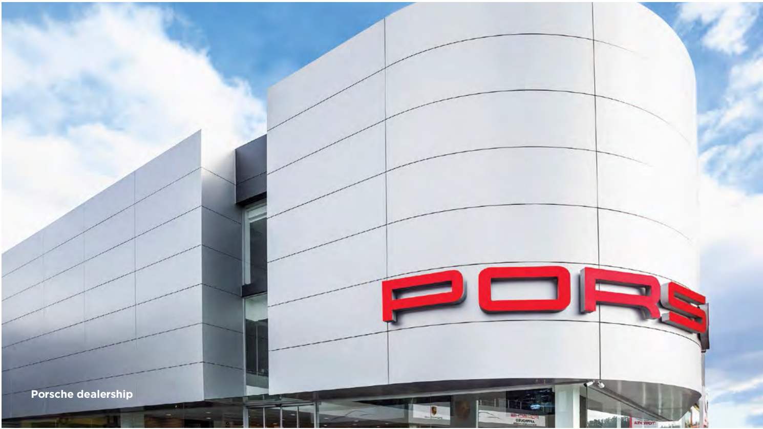
Porsche Car Dealer A Coruña, Spain 2017 Finish: Silver metallic Material: Stacbond FR System: STB-CH Transformation: Bending with rollers
