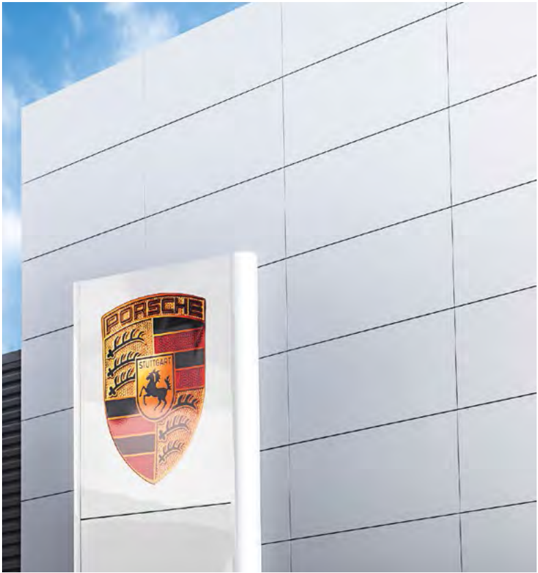
Porsche Car Dealer A Coruña, Spain 2017 Finish: Silver metallic Material: Stacbond FR System: STB-CH Transformation: Bending with rollers
