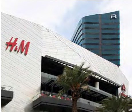
Fashion Drive shopping centre Monterrey, Mexico 2018 Finish: Golden pearl Material: Stacbond FR System: Ad-hoc Transformation: Bending with rollers
